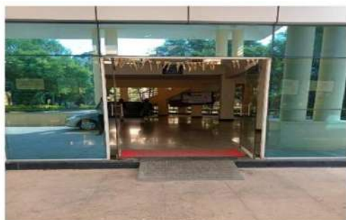
BARRIER FREE ENVIRONMENT- MAIN BLOCK RAMP
